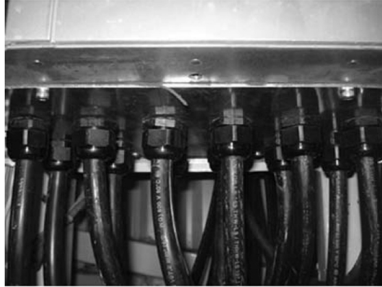
Figure 37: Example of proper installation of the connector plate
