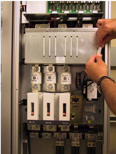
Illustration 3.4 Reconnecting Fan Transformer Wiring
