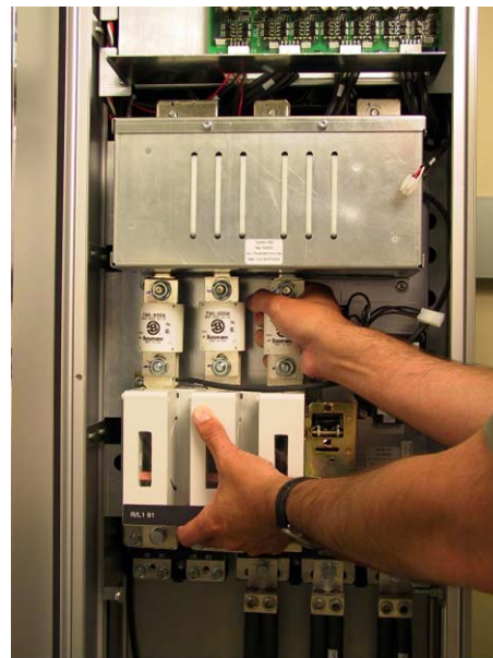
Illustration 3.3 Input Plate with RFI, Disconnect and Fuses
