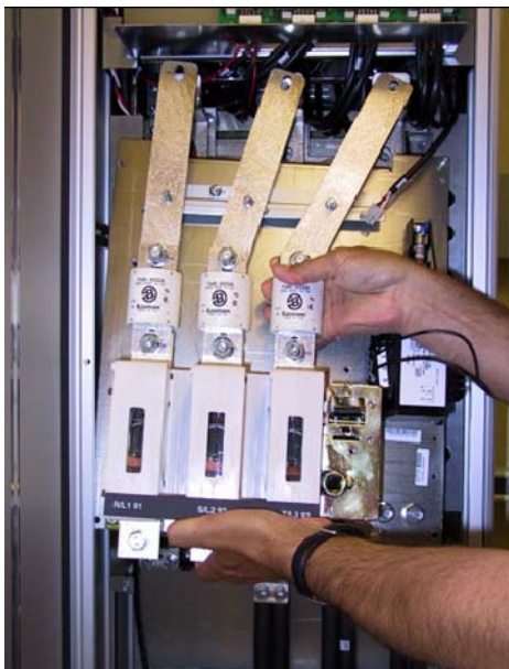
Illustration 3.1 Align the Input Plate with Studs. Fused Disconnect Configuration Shown.
