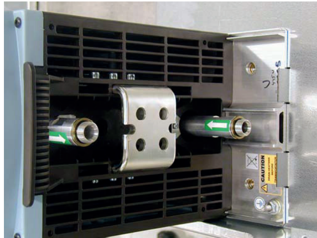
Figure 27. Aluminium hose adapters
