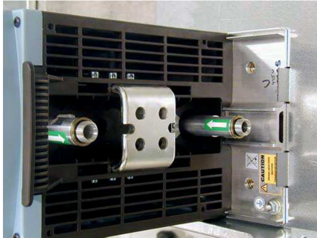
Figure 27. Aluminium hose adapters
