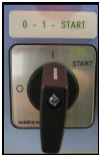
Figure 26. 0-1-Start Control switch (-S10)
