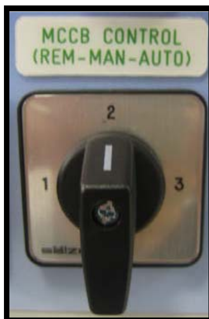
Figure 25. MCCB Control selector switch (-S6)
