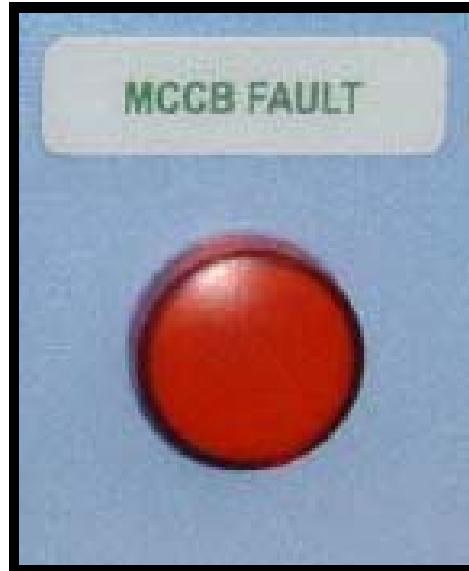
Figure 29. MCCB FAULT indicator
