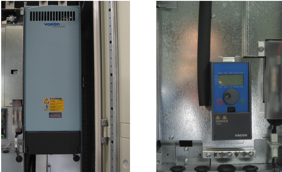
Figure 5-4. Mounting of the control unit.
