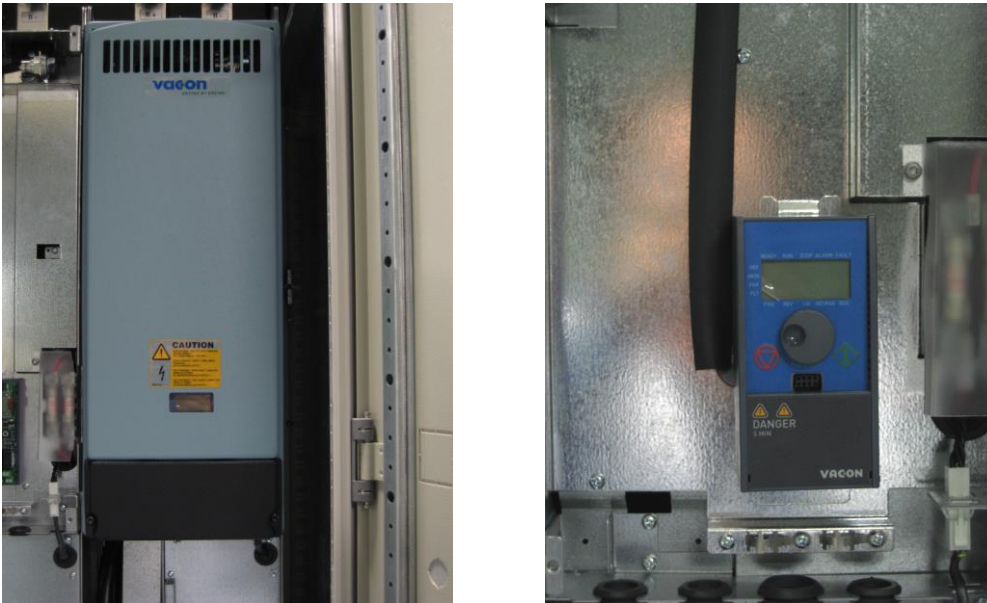
Figure 5-4. Mounting of the control unit.
