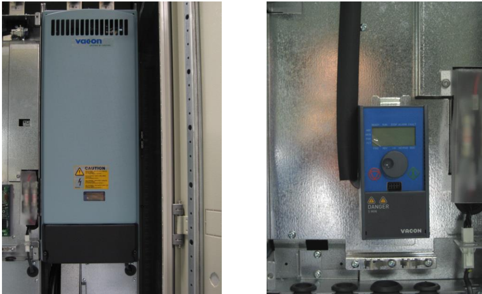
Figure 5-4. Mounting of the control unit.
