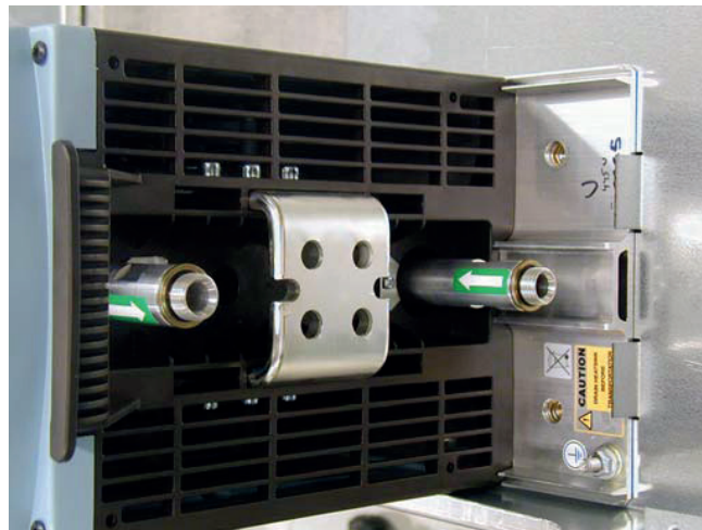
Figure 27. Aluminium hose adapters
