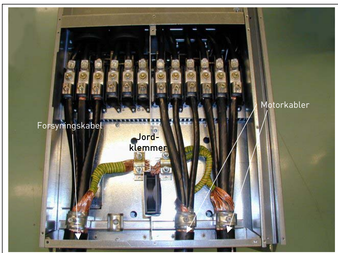
Figur 6-15 Installation af kabler i Vacon NX, FR9
