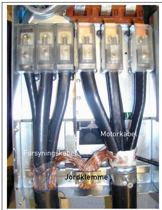
Figur 6-12. Installation af kabler i Vacon NX, FR8
