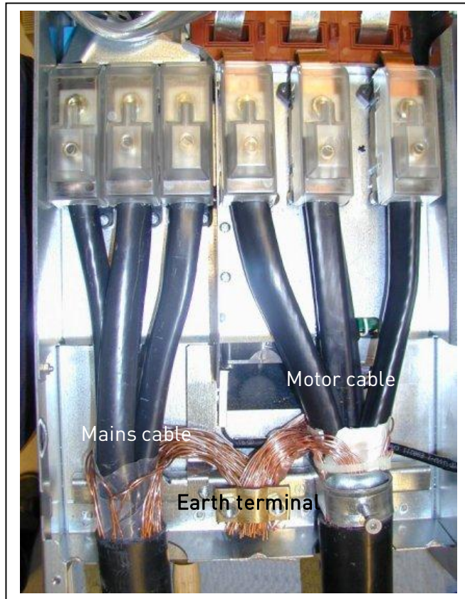
Figure 6-17. Cable installation in Vacon NXS/P, FR8
