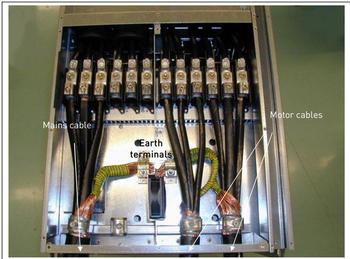
Figure 6-20. Cable installation in Vacon NXS/P, FR9
