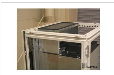
Illustration 3.46: Top duct installed
