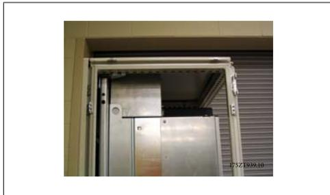
Illustration 3.38: Top duct work and enclosure top installed
