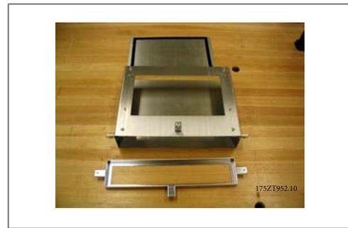
Illustration 3.52: Bottom ductwork partially assembled
