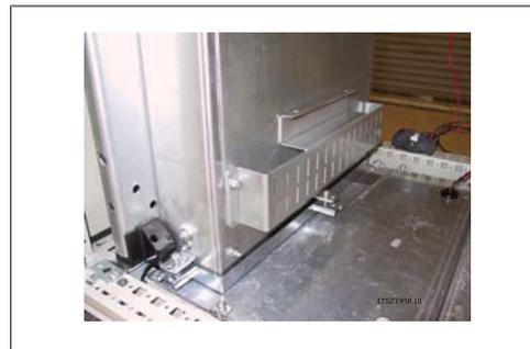
Illustration 3.59: Bottom duct installed.
