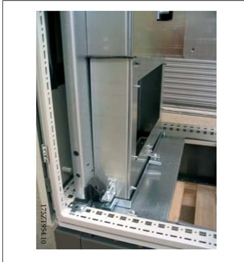
The cutout is made on the innermost gland plate. The remaining two gland plates must be removed for the installation of the bottom duct assembly.
