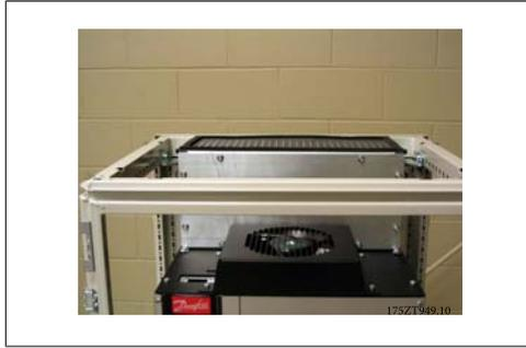
Illustration 3.48: Top duct closing plate installed
