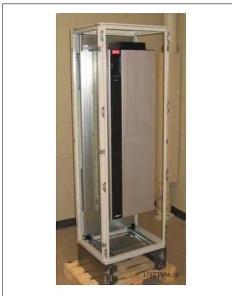
Illustration 3.36: Frequency converter installed in cabinet
