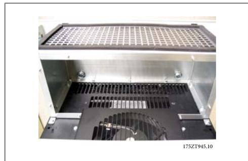
Illustration 3.42: Top duct installed
