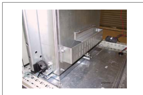
Illustration 3.59: Gaine inférieure installée
