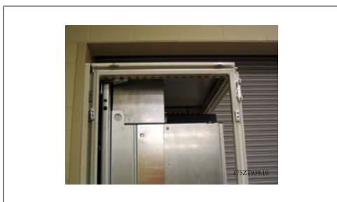
3.38: Top duct work and enclosure top installed
