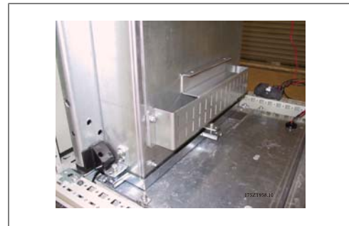
3.59: Bottom duct installed.
