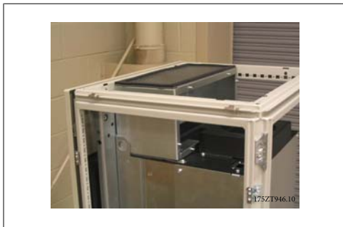
3.46: Top duct installed
