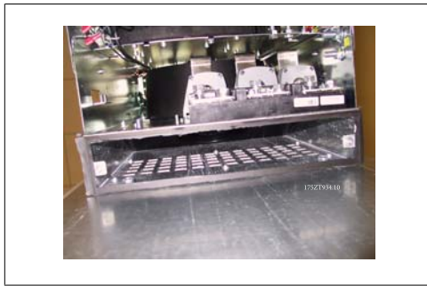
3.33: Bottom duct adapter installed
