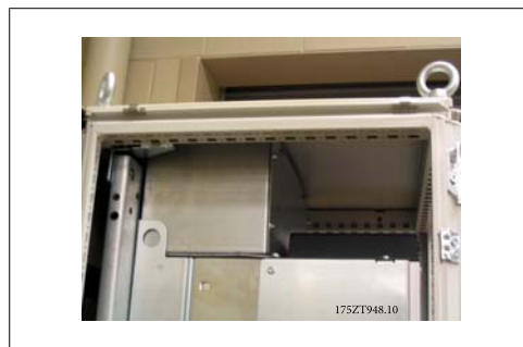
3.49: Enclosure top installed
