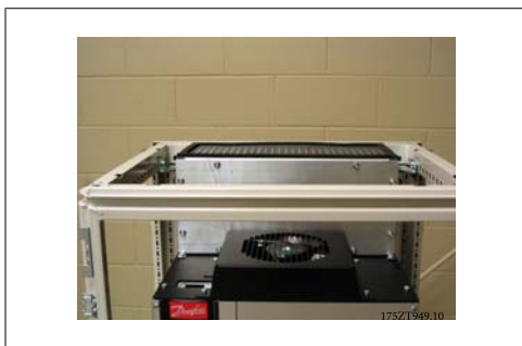
3.48: Top duct closing plate installed
