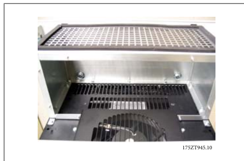
Illustration 3.42: Top duct installed
