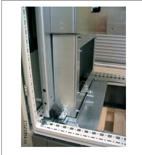
Illustration 3.54: Temporarily install duct work to mark cutout on the gland
