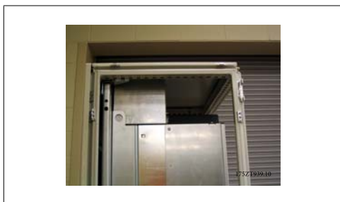
Illustration 3.38: Top duct work and enclosure top installed
