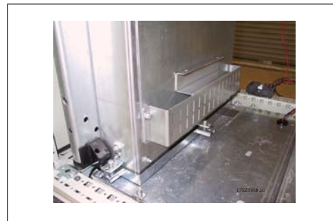
Illustration 3.59: Bottom duct installed.
