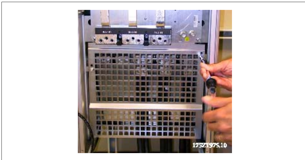
Illustration 3.81: Mounting of EMC shield.
