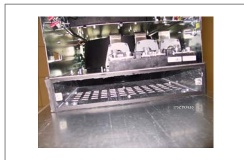
Illustration 3.33: Bottom duct adapter installed
