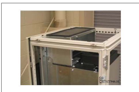
Illustration 3.46: Top duct installed
