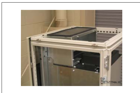
Illustration 3.46: Gaine supérieure installée
