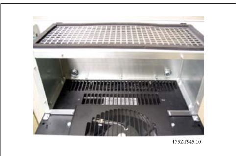
Illustration 3.42: Gaine supérieure installée
