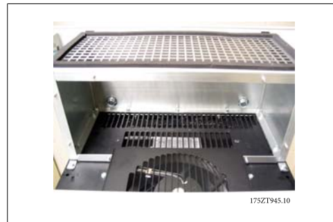
3.42: Top duct installed
