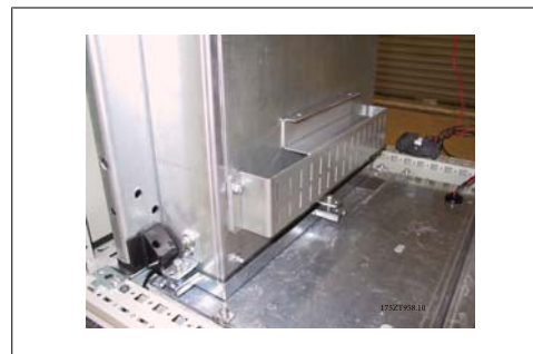
3.59: Bottom duct installed.
