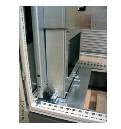
3.54: Temporarily install the duct work to mark the cut-out on the gland.
