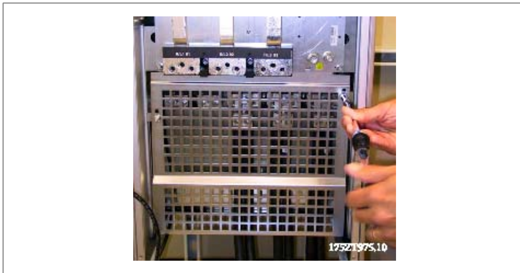
3.81: Mount the EMC shield.
