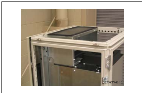
3.46: Top duct installed
