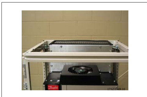
3.48: Top duct closing plate installed
