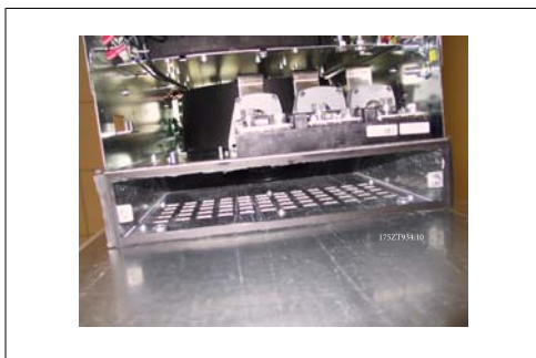
3.33: Bottom duct adapter installed
