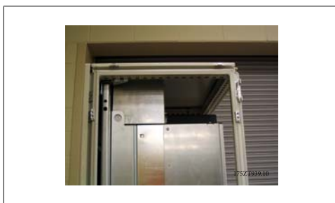
3.38: Top duct work and enclosure top installed
