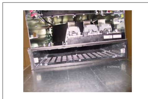
Illustration 3.33: Bottom duct adapter installed
