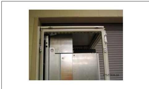
Illustration 3.38: Top duct work and enclosure top installed
