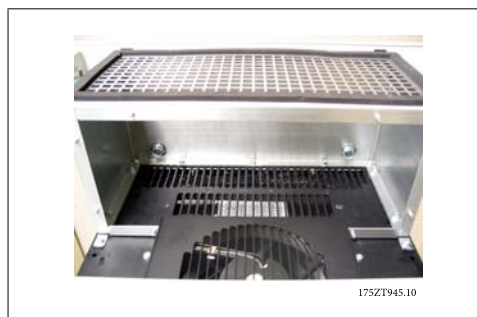
Illustration 3.42: Gaine supérieure installée
