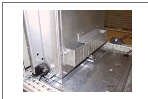
Illustration 3.59: Gaine inférieure installée
