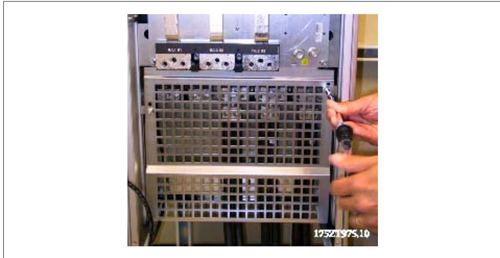
3.81: Mount the EMC shield.
