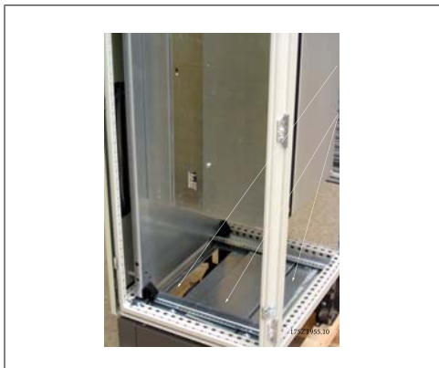
3.55: Enclosure bottom cut-out
