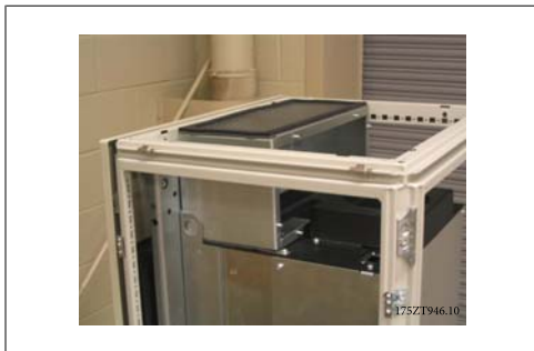
3.46: Top duct installed
