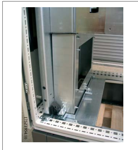
3.54: Temporarily install the duct work to mark the cut-out on the gland.
