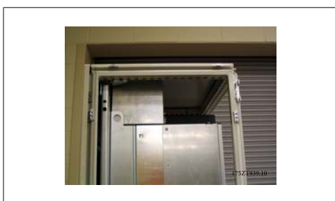
3.38: Top duct work and enclosure top installed
