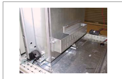
3.59: Bottom duct installed.
