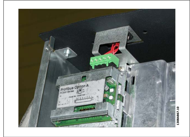
Figure 3.49: Top connection for the serial communication bus.
