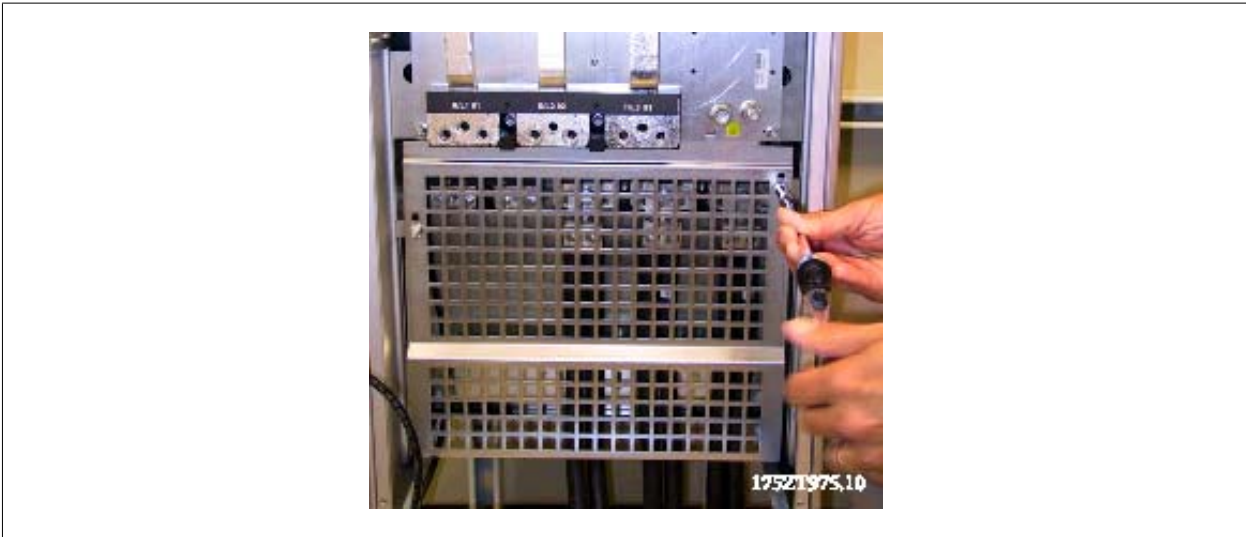
Figure 3.47: Mount the EMC shield.
