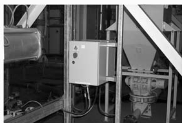
Illustration 1.14: Gammel løsning: Motorregulator - tavle monteret decentralt
