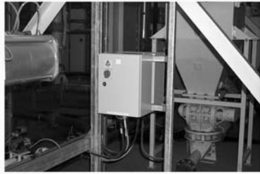
Illustration 1.14: Old solution: Motor control - panel mounted decentrally
