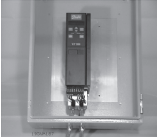
Figure 7 Complete VLT 2800 Cold Plate Installation
