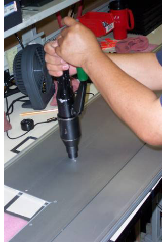
Photo 14. Drilling and punching the door to install disconnect han-
