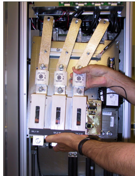
Photo 8. Installing of kit containing Disconnect and Fuses
