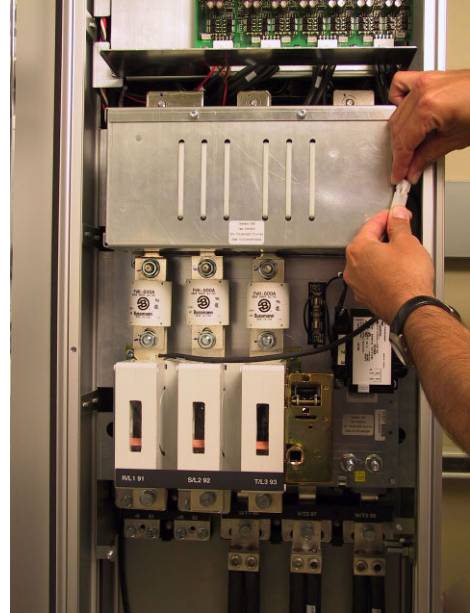
Photo 11. Reconnecting Fan Transformer Wiring
