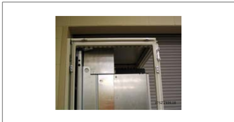
Illustration 4.10: Top duct work and enclosure top installed
