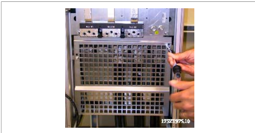
Illustration 3.39: Mounting of EMC shield.
