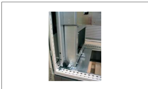
Illustration 4.26: Temporarily install duct work to mark cutout on the gland
