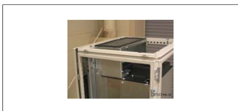
Illustration 4.18: Top duct installed
