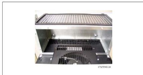
Illustration 4.14: Top duct installed
