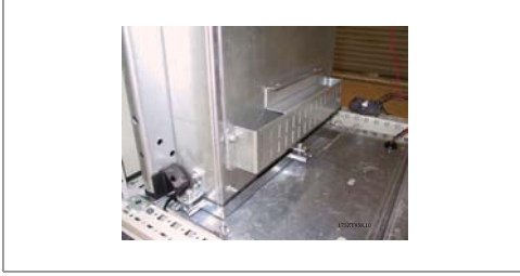
Illustration 4.31: Bottom duct installed.
