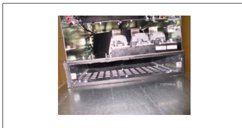
Illustration 4.5: Bottom duct adapter installed
