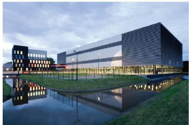
Equinix Data Centre in the Netherlands, protected with SEM-SAFE® high-pressure water mist system
