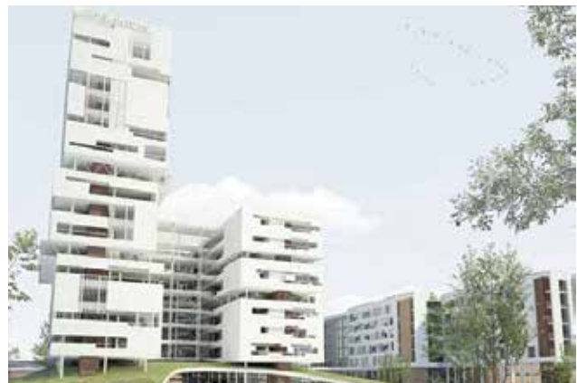
DNU Skejby University Hospital in Denmark
