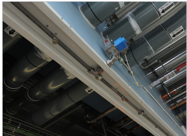
The innovation behind SEM-SAFE® has allowed for water curtains to replace traditional fire doors.
