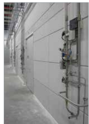
Danfoss Semco pre-action section valve placement in Equinix AM3
