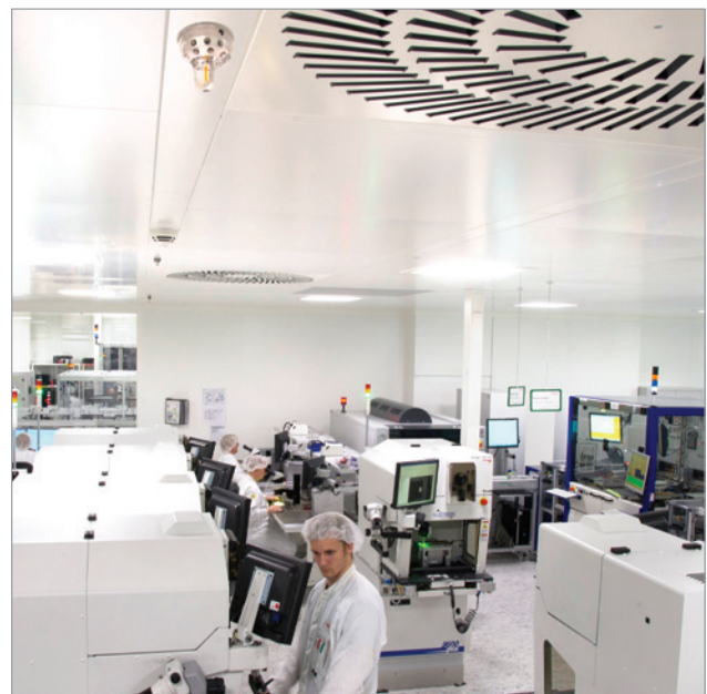
SEM-SAFE® nozzle installed in the clean room at Danfoss Silicon Power
