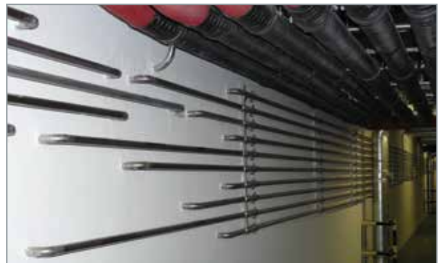
High quality stainless steel pipe offers long life span, while the small pipe dimension ensures easy installation and integration as well as an aesthetic design
